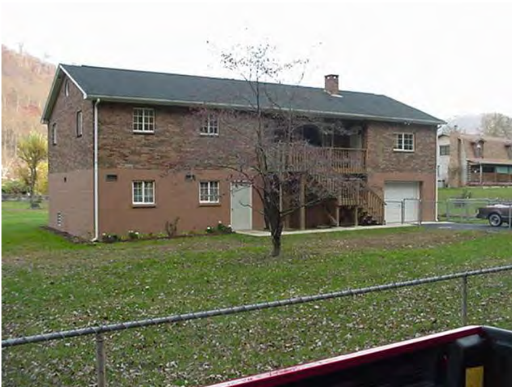
Figure B-5. Example of a house raised on a closed foundation.
