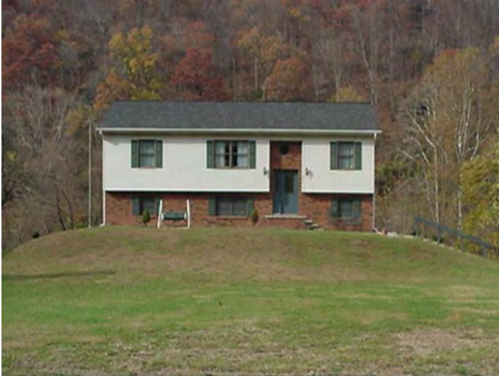
Figure B-6. Example of a house raised on fill.
