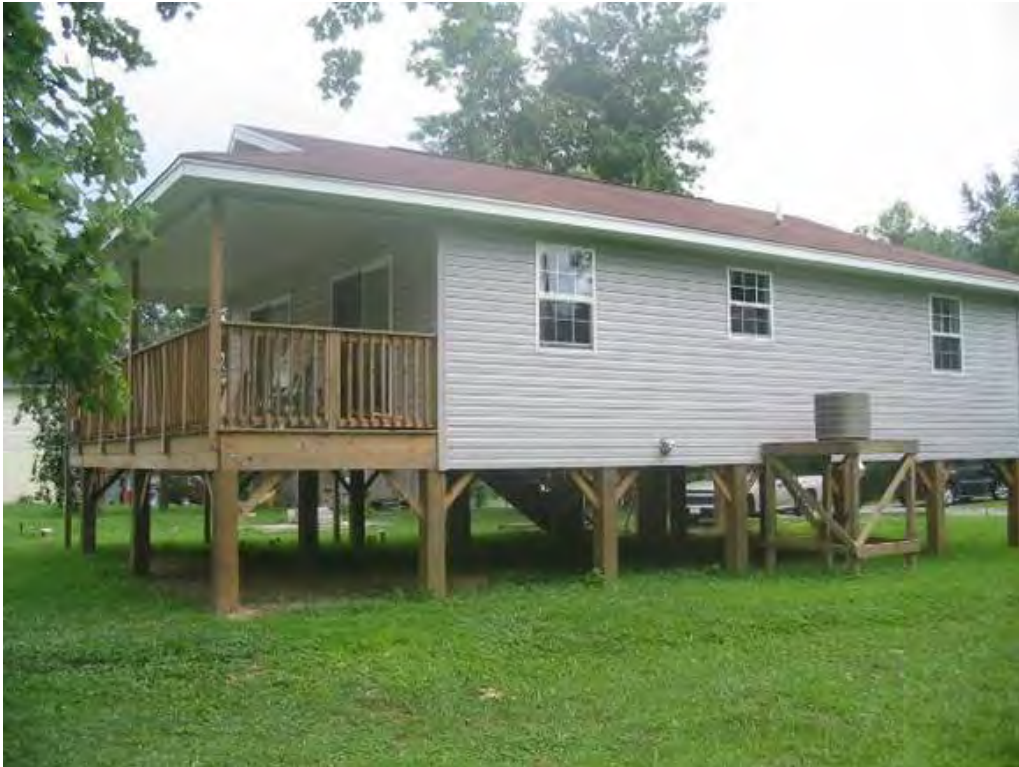
Figure B-4. Example of a house raised on an open foundation.
